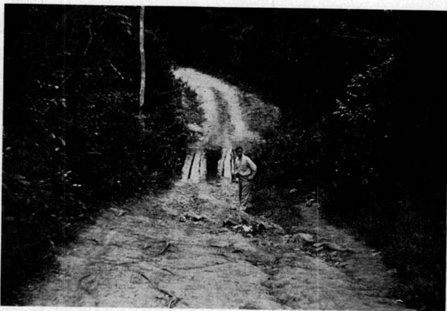
Fig. 3.—Old road to Itapací, now unmaintained and little used. The vegetation is denser in this small valley than along most of the route which goes through savanna. The rude bridge of hewn logs imbedded and retained only by earth fill was typical of the first road to serve Itapací.
