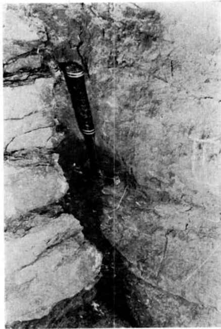
FIG. 6.—Close-up view of filled joint (Site 2). Pick at contact of gray-brown pebbly clay above and reddish-brown silty clay below.
