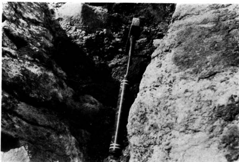
FIG. 4.—Close-up view of filled joint (Site 1). Pick at contact of Champaign till above and plastic clay below.
