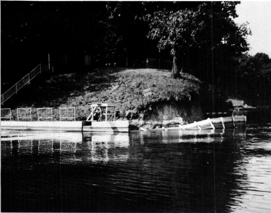
FIGURE 4. Inadequate barrier fails to stop bank erosion.
