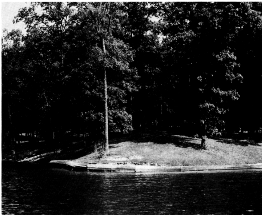
FIGURE 5. Wood barrier uprooted by high water.
